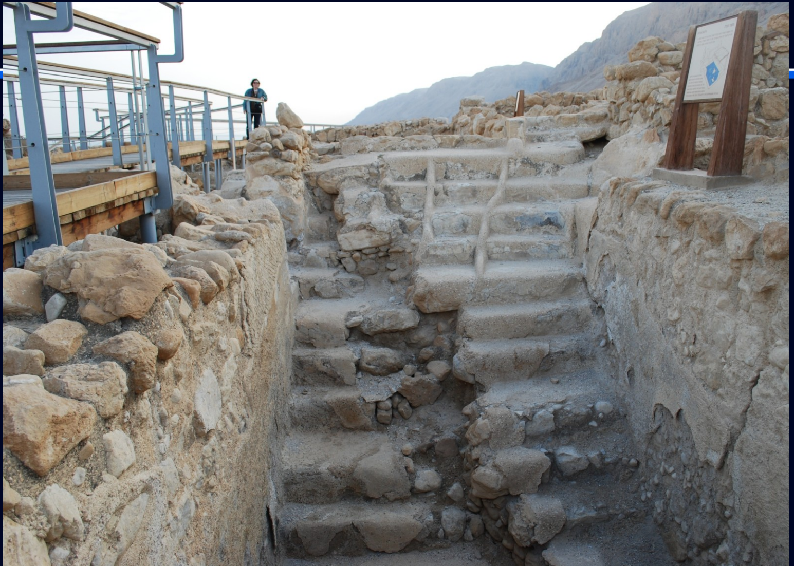
Faulting cuts architecture at Qumran. 31 B.C. displacement is mostly dip-slip.
